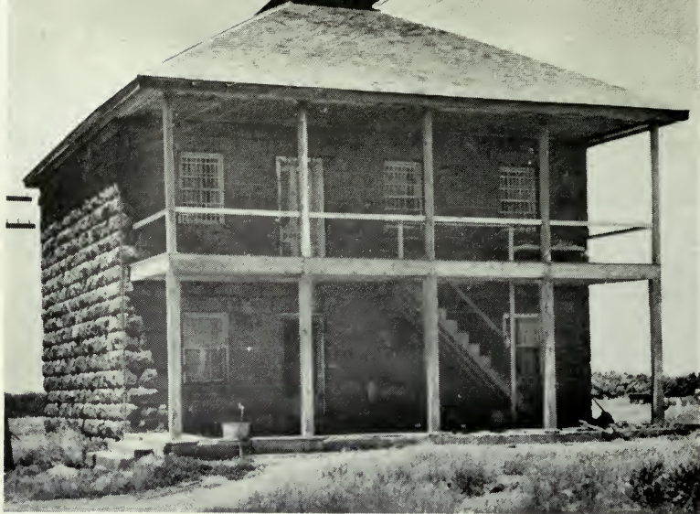
Fort Harker guardhouse, Kanopolis.
